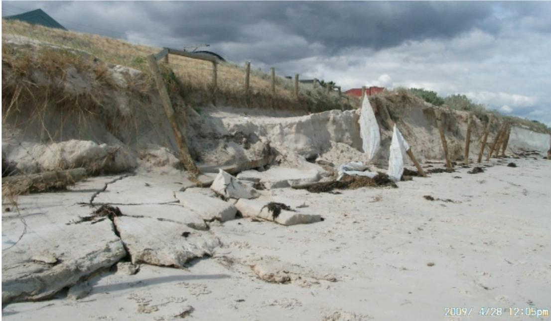
Figure 46: Storm damage at coast at Hillview St 2009; the consolidated path to the beach has been broken into slabs, each acting like a mini rocky shore.
